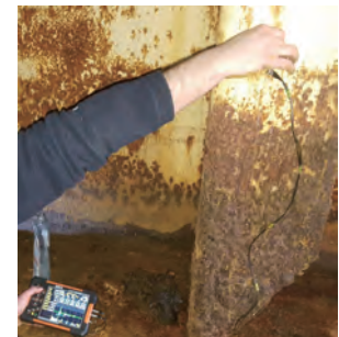
Port dock thickness measurement
